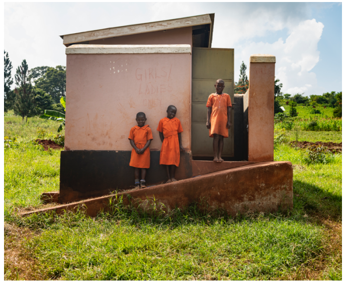
A new block of toilets at primary school in Kinoni.
